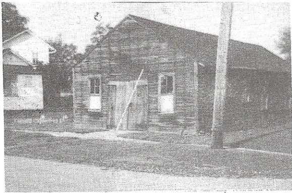
Old Blacksmith Shop
